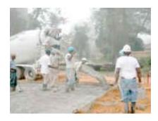
A typical mix of cement, sand and stones is written as a ratio, such as 1:2:6.
